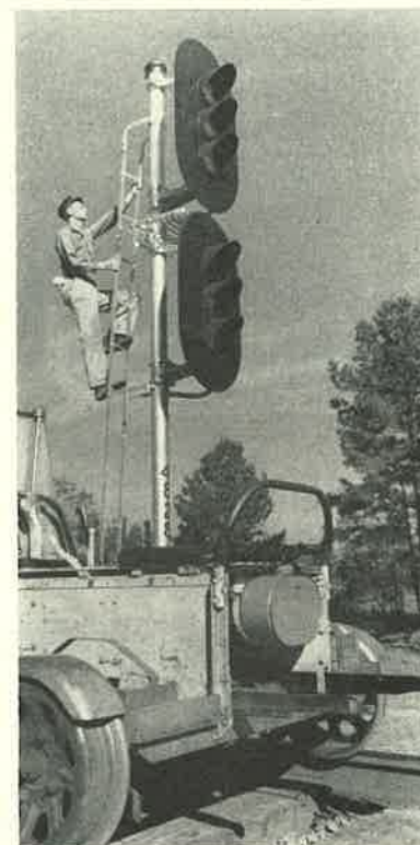
A Signal Maintainer on the Job
