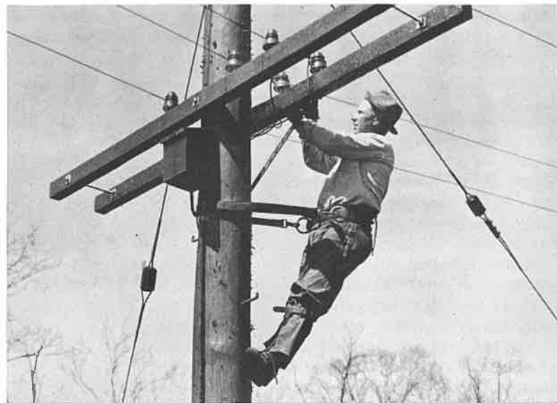
Lineman Repairing Communication Lines
