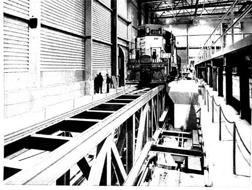
WHEEL TRUING TABLE — Workers prepare a diesel to undergo repairs on a unique dual wheel truing machine that will true two axles simultaneously. Currently, only one wheel
