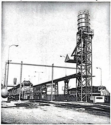
REFUELING — New fueling facilities are located directly northeast of the main shop building. It consists of four 500-foot long service tracks equipped with two servicing manifolds, inspection pits and two gantry type sanding cranes.
