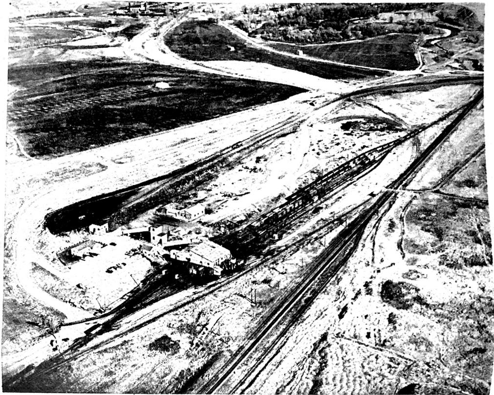
**LOADING DOCKS** — Aerial photo of the Big Horn Coal Company at Sheridan, Wyo., shows the tipples and railroad car loading facilities near the huge mine.
